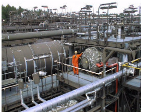
Figure 6. General view of the separator
